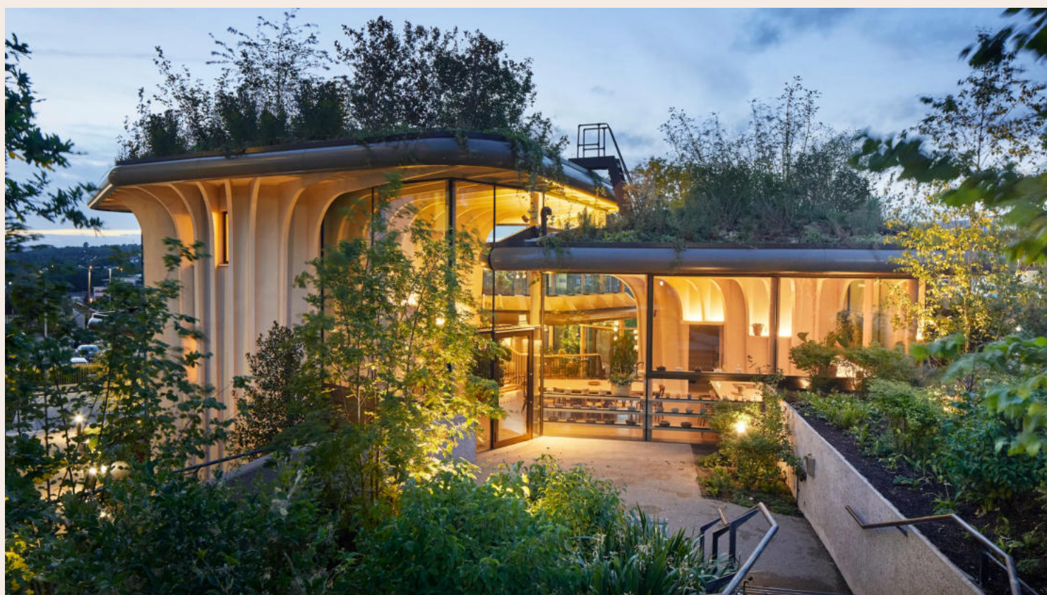
Verdant Maggie's Centre, Leeds, England
