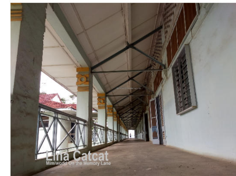
OPENING CONCRETE PARAPETS ABOVE ON THE WALL
