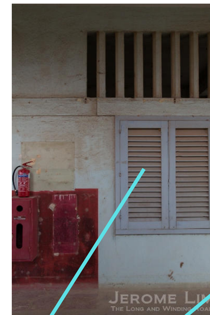
Louvred doors and windows
