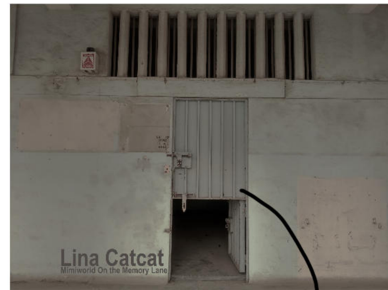
ARMOURY STOREROOM ENTRANCE
