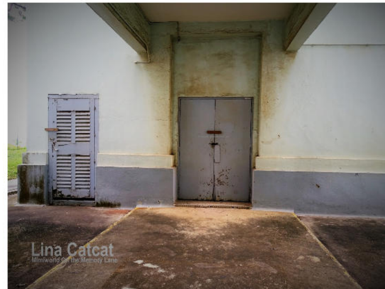
TOILET AT GROUND FLOOR SERVICE BLOCK
